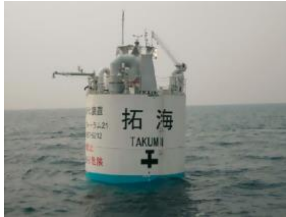
Fig. 7 Photo of OTEC in operation
