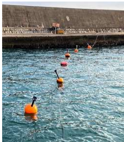
Fig.6 Installed in the sea
