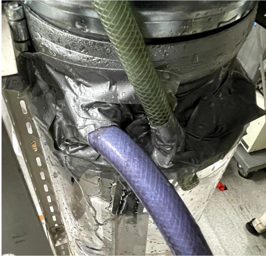
Figure 59 Gap sealed state (The left side is the water supply hose)
