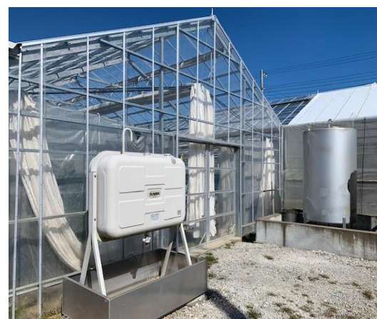
Kerosene tank (bottom left), carbon dioxide tank (back right)
