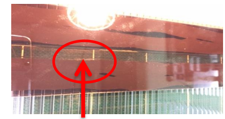
*Silicone is just at the waterway line. The trick is to extend it to
